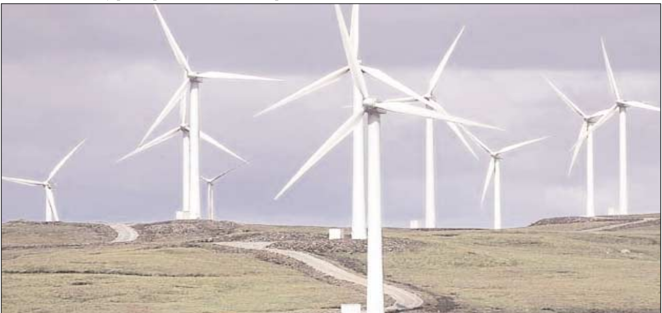
ScottishPower's 30MW Beinn an Tuirc wind site in Argyll, opened in 2001 by then Energy Minister Brian Wilson.
