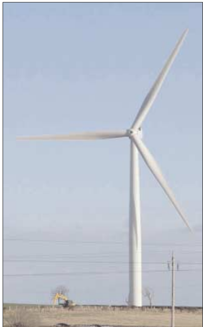
AMEC's 3-turbine site at Elwick, near Hartlepool. The nearby digger suggests the scale (2.75MW NEG Micon, 100m tip ht.)
